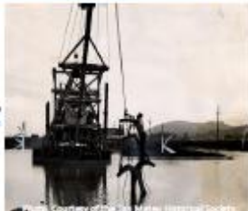
Newsstory: Dredge works to protect San Mateo "Seal Slough Drainage Project" Under Way." JAN
